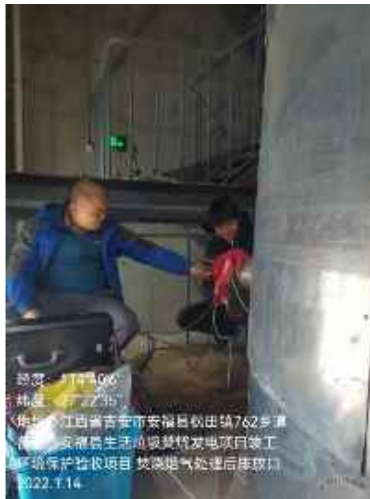
焚烧烟气处理后排放口②
